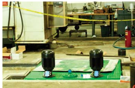
In-Ground Dirty Pump-Back Sump System Pit Installed with Closed Piping Returns.
