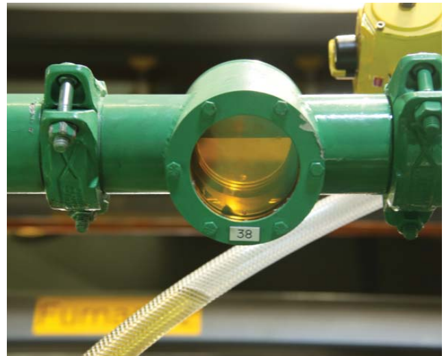
Hot Quench Oil Filtered to Below 5 Microns Clarity.
