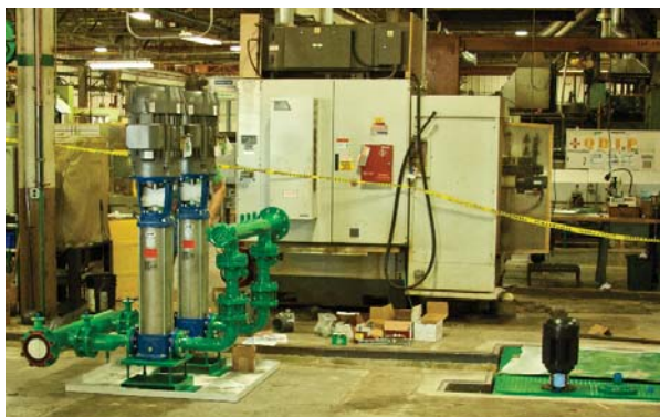
In-Ground Dirty Pump-Back Sump Return System with Standby Pump.
