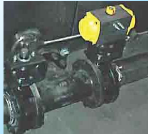
3-Way Valve Assembly for Positive Vacuum Break
